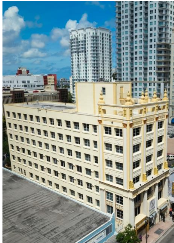
Building at present, following post-hurricane reconstruction
