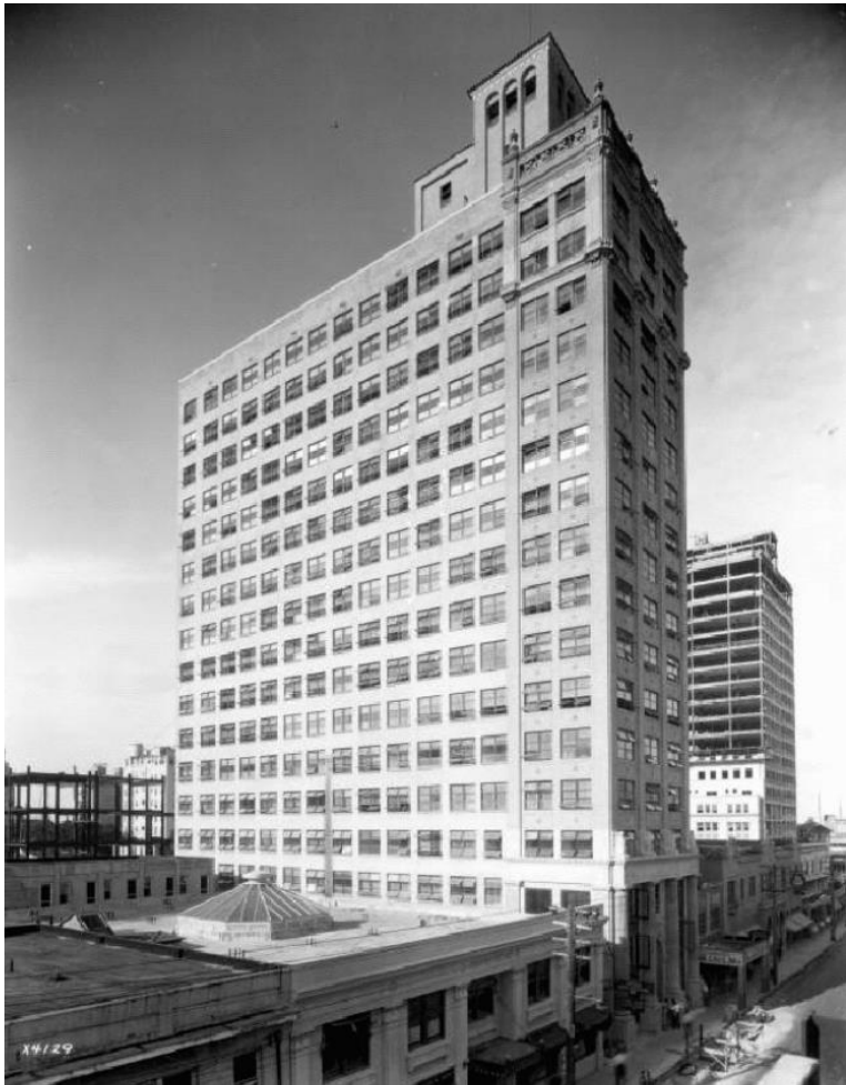
Building as constructed in 1925 (South Florida Business Journal)
